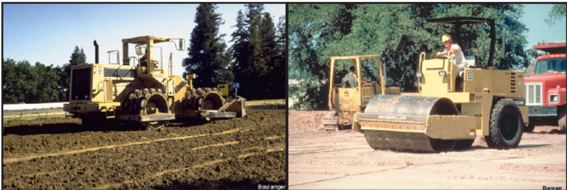
Fig. 1: Field Compaction using a Sheepsfoot Compactor.
